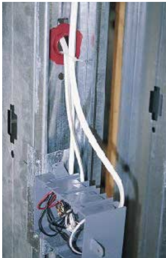
Figure 5. Plastic grommets protect wiring from the sharp edges of the framing punchouts. At electrical boxes, the wiring is secured to a special connector screwed to the stud (above), or a plastic wire tie looped through a punchout (right).
