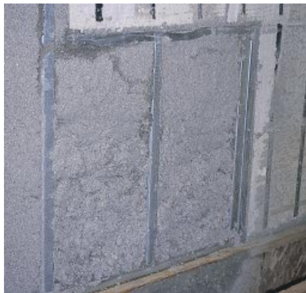
Figure 8. Spray cellulose in stud cavities reduces sound transmission and provides backing for 5/8 inch drywall.
