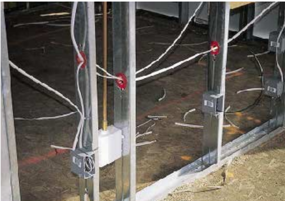
Figure 5. Plastic grommets protect wiring from the sharp edges of the framing punchouts. At electrical boxes, the wiring is secured to a special connector screwed to the stud (above), or a plastic wire tie looped through a punchout (right).
